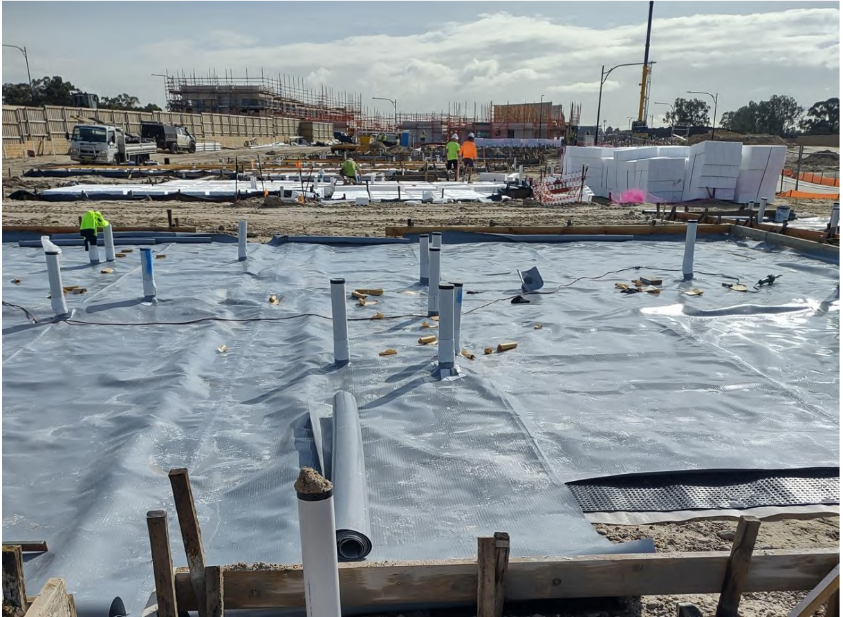
Figure 3: Welded membrane
