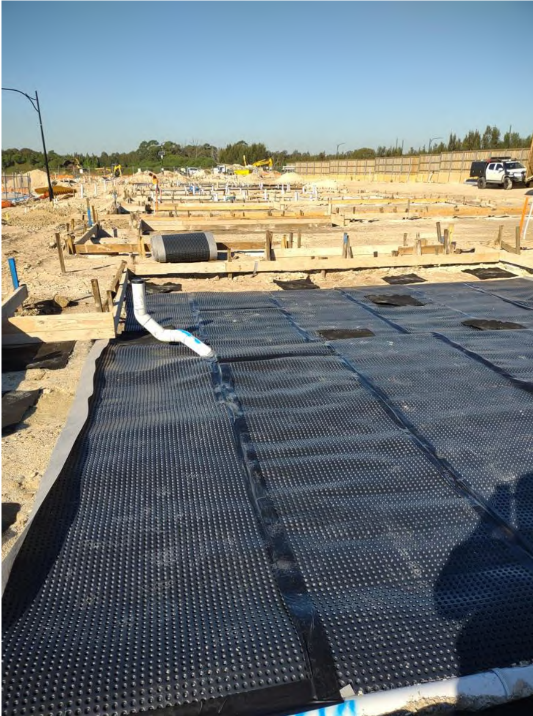
Figure 2: Gas drainage layer
