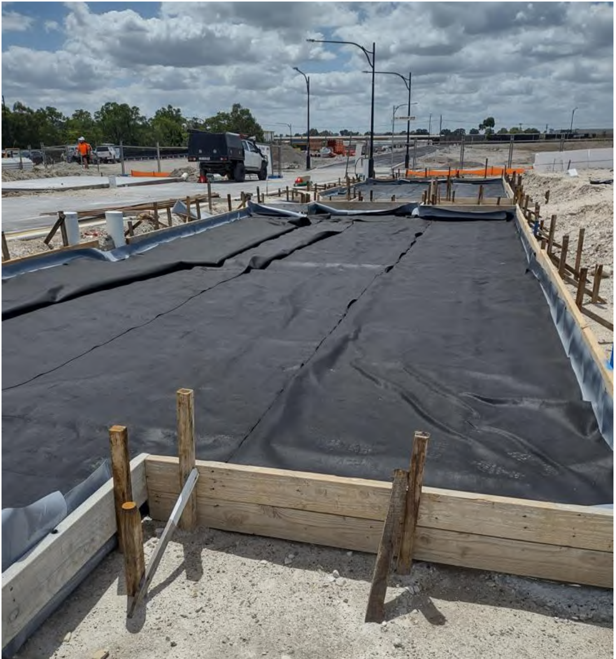
Figure 4: Geotextile protection layer
